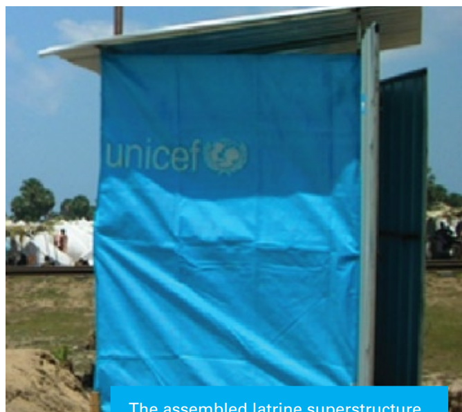
The assembled latrine superstructure
