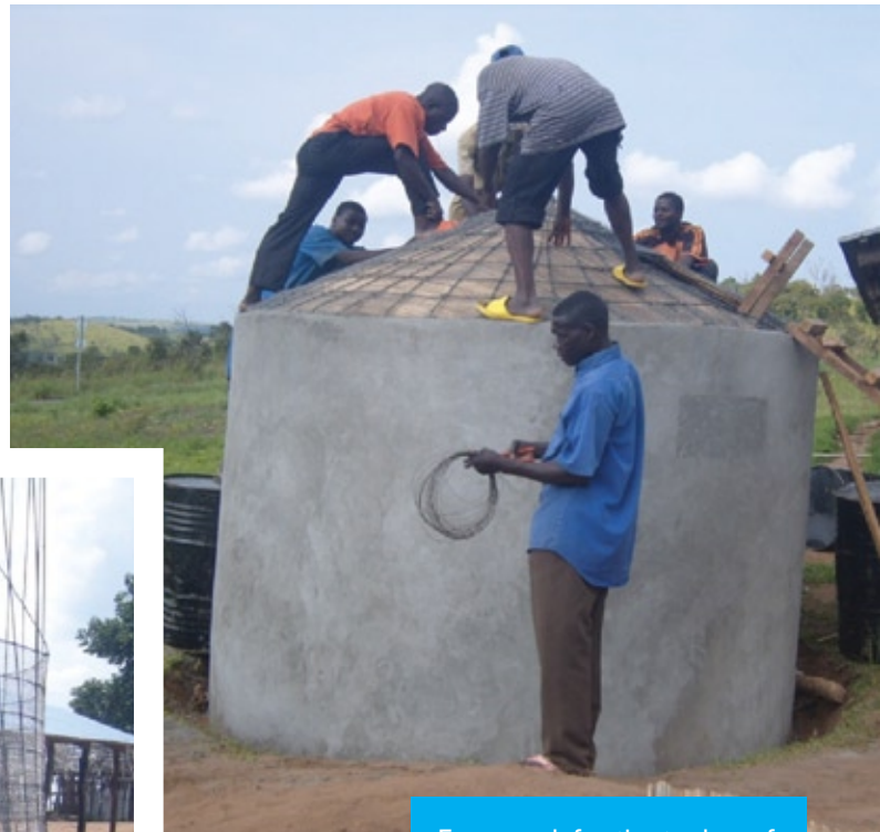
Formwork for the tank roof
