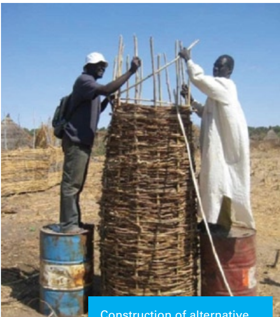
Construction of alternative (from sand bags) pit liner for sandy soils
