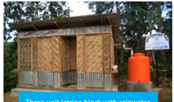
Three-unit latrine block with rainwater harvesting system
