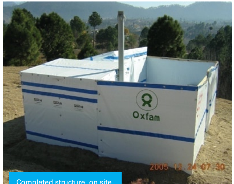
Completed structure, on site
