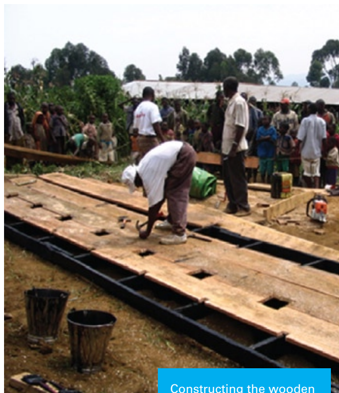
Constructing the wooden floor for a latrine block
