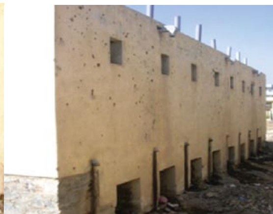
At Rahman Meena School, Kabul City, vault latrines were observed to be open in the back and without doors; waste material was flowing out of the latrines.
