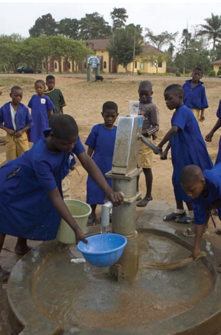
Students use a Mark II-type handpump at a primary school in Araromi Oke Village, south-western Nigeria.
