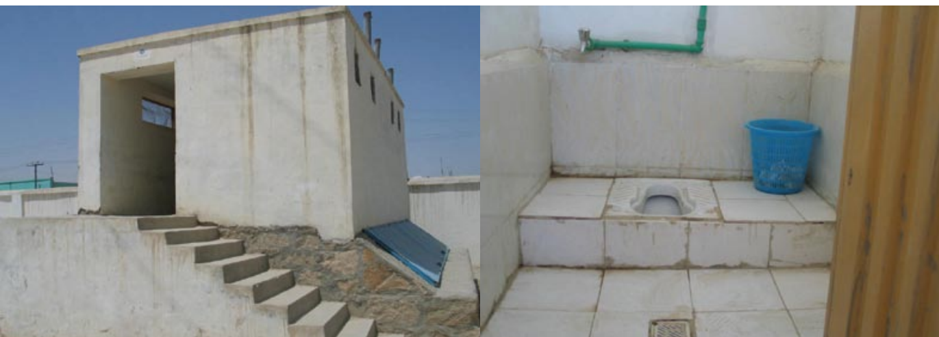
Old single-vault latrine after conversion to pour flush, Raies Abdul Khaliq school, Mazar.
