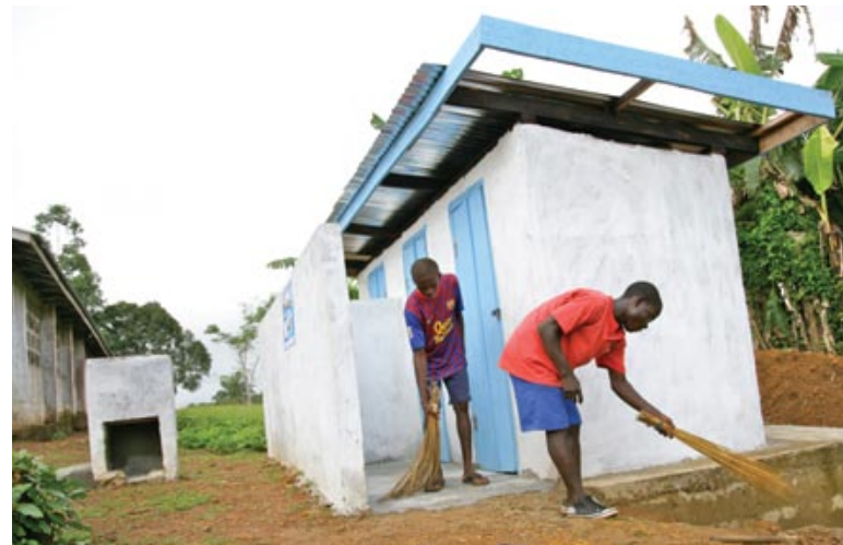
Students help keep the newly built latrines clean at a school in north-eastern Liberia.
