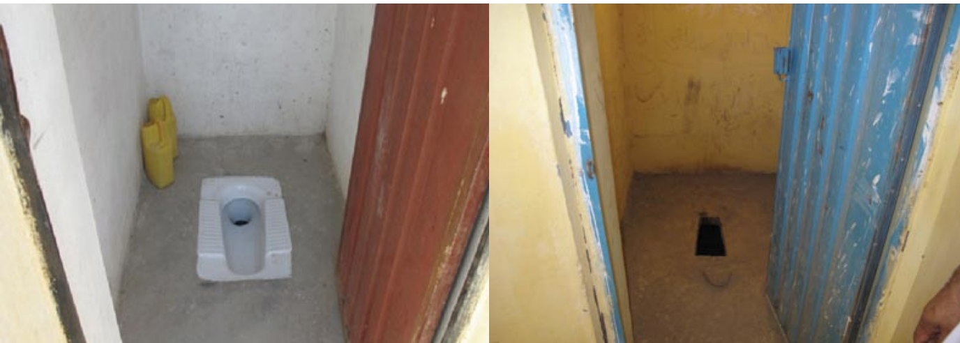
Flush toilet connected to a septic tank at a school in Hashim barat ( left ) and a latrine at Tajrbawei.
