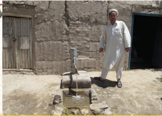
Hand-washing facility in Fatima Auz ahar, with only one out of five faucets working (left) and the handpump at a school in Said Abad, with unclean area around the water point and a broken apron and drainage channel.
