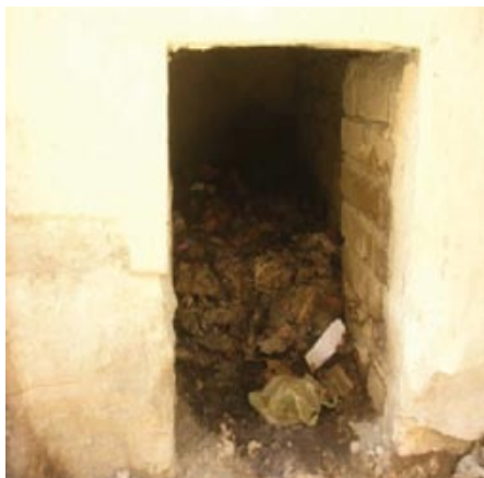
At Rahman Meena School, Kabul City, vault latrines were observed to be open in the back and without doors; waste material was flowing out of the latrines.
