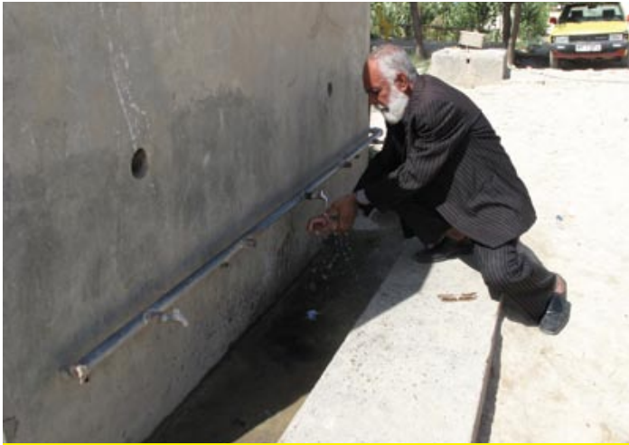
Hand-washing facility in Fatima Auz ahar, with only one out of five faucets working (left) and the handpump at a school in Said Abad, with unclean area around the water point and a broken apron and drainage channel.
