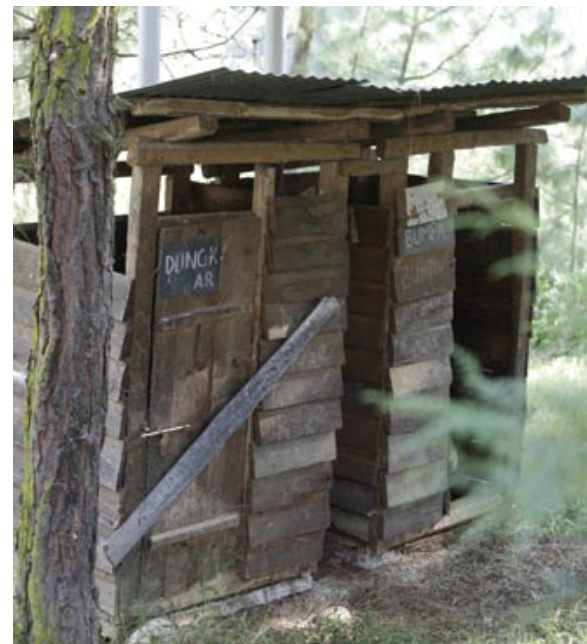
Toilets built with local materials.
